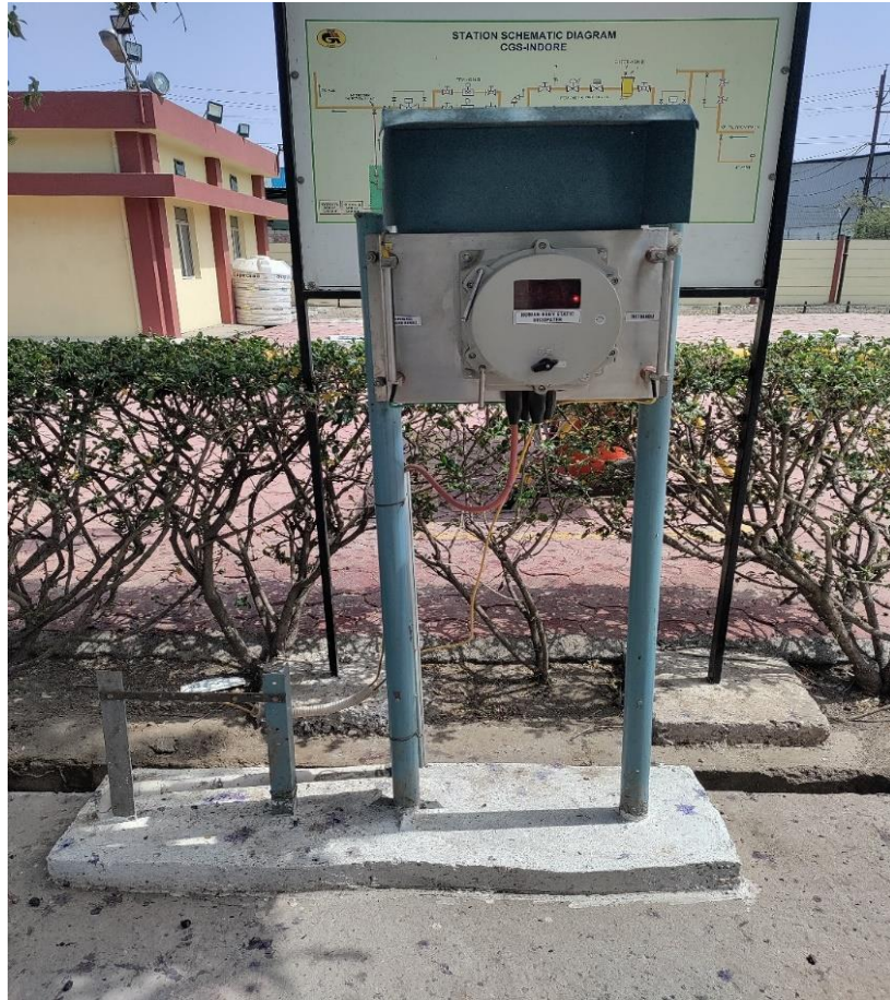
Human Body Static Dissipater provides a simple display indication if the resistance is above or below the value set in the unit
