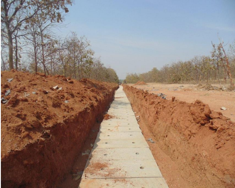
Concrete Slabs – Future Development Areas
