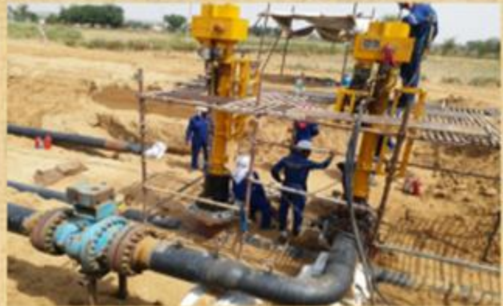
HOT TAPPING IN PROGRESS
