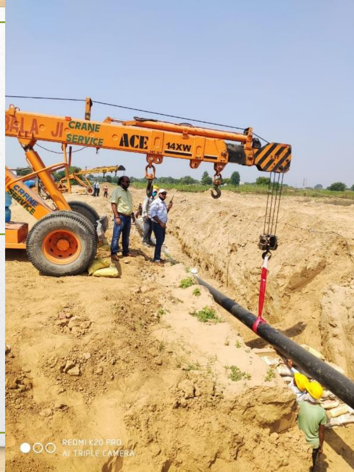
Lowering under progress
