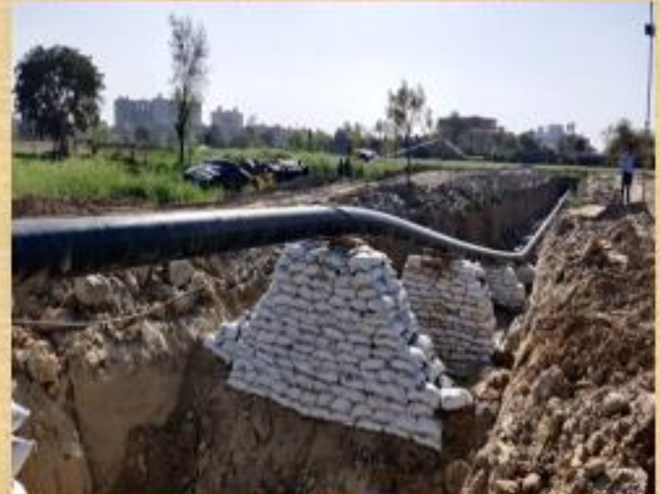
Lowering under progress
