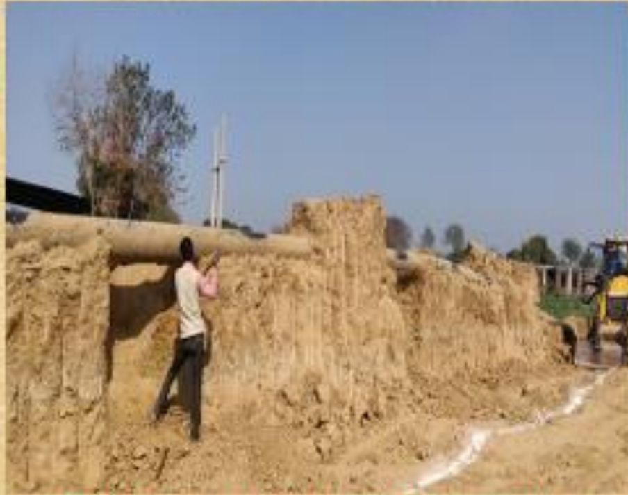
P/L Position before Lowering (CH. 1172.80 KM)
