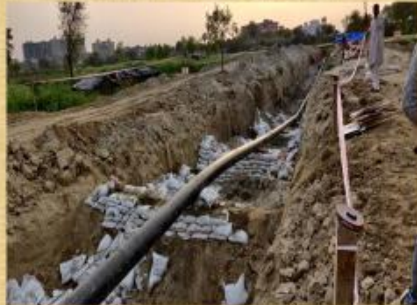
Final position after lowering
