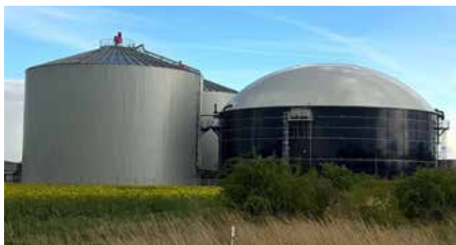
CBG Plant at Namakkal, Tamil Nadu
