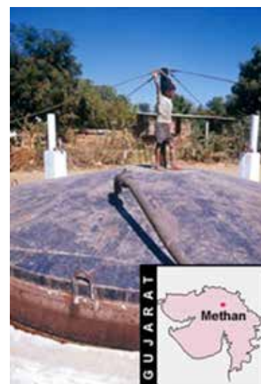
Methan Village Biogas Plant
