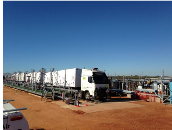
Virtual CNG Pipeline
