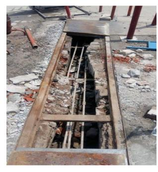
At retail outlets, movement of heavy vehicles Trucks Gas tubing trenches are getting damaged.
