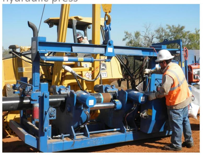
Zap Lok installation 7: move machine to next joint
