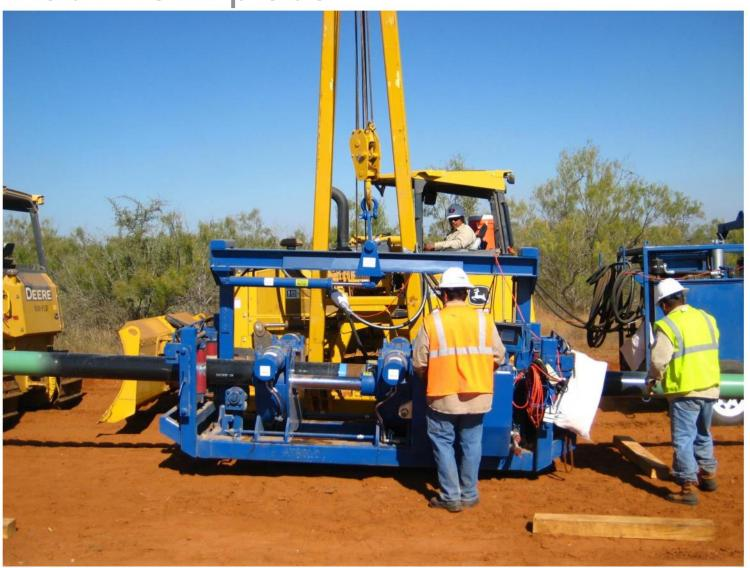
Zap Lok installation 6: make up joint with hydraulic press
