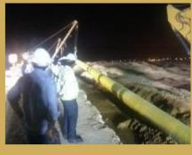
Saudi Aramco needed to protect hundreds of feet of new 24" pipeline during the HDD pull back which would pass through aggressively rocky terrain that could possibly damage the pipe's coated surface and cause premature coating failure.
